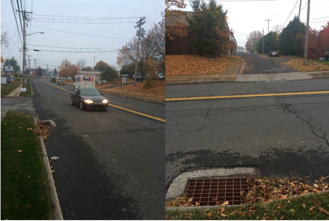
282 Woodmont Road looking north
