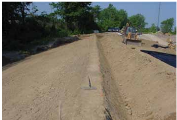
Proper excavation, grading and compaction is critical to the performance of the ACB system.
