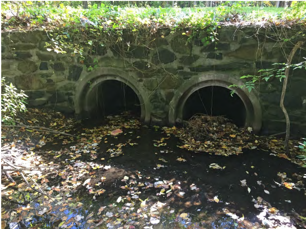
Twin 42" RCP culvert at Pepes Farm Road
