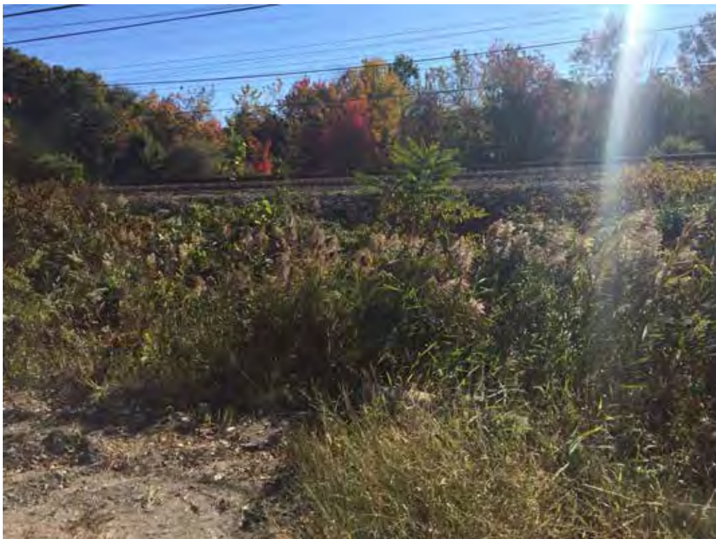
Upstream Railroad Embankment at Culvert
