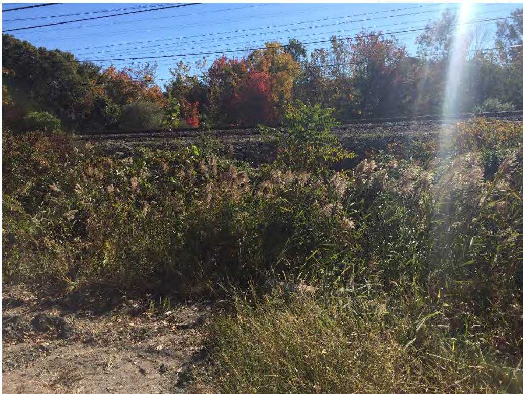
Upstream Railroad Embankment at Culvert
