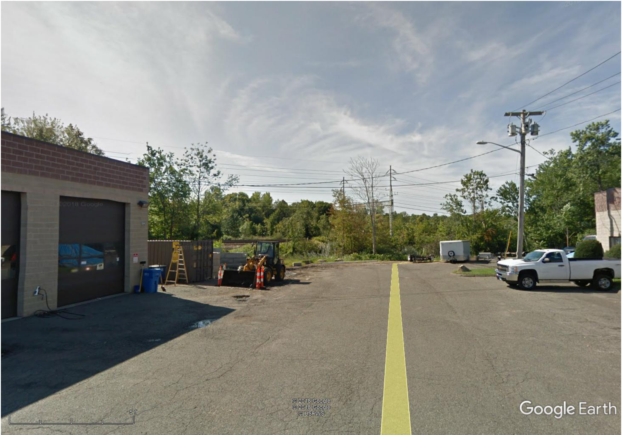
View of the general area for staging at the inlet end of the railroad culvert.
