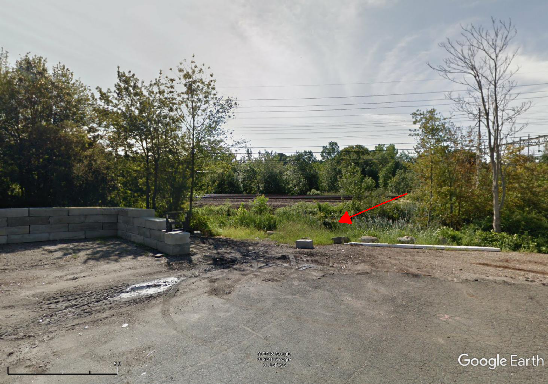
View looking at the inlet side work area. Red arrow indicates the approximate location of the inlet headwall.
