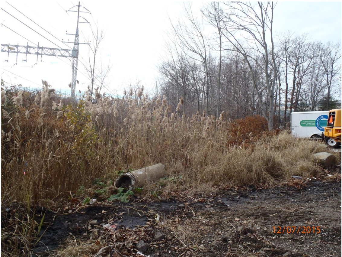
5. Upstream Side Looking West
