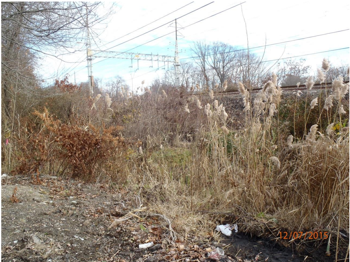
6. Upstream Side looking East
