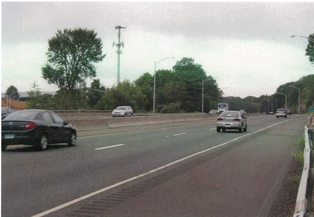
4. Southbound Lanes Looking West across Bridge
