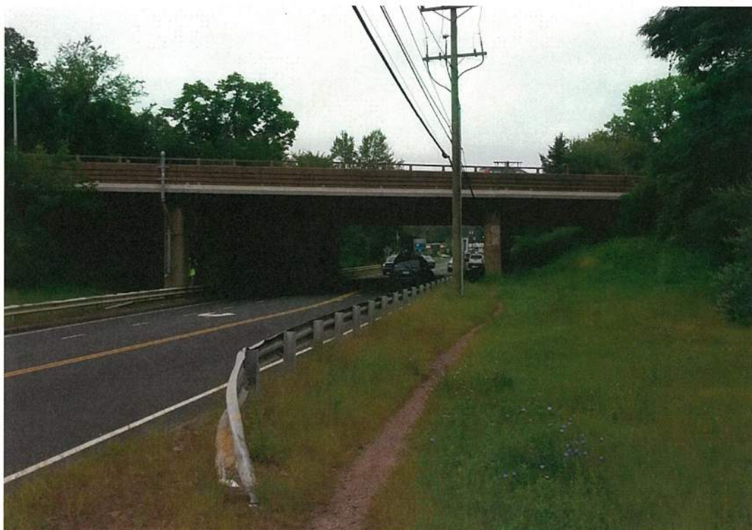
2. South Elevation (Note: View is looking Northbound on Route 1)
