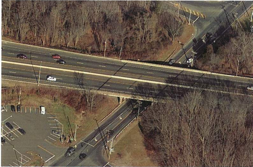
Image 1: Bridge #00196. Image courtesy of Bing Maps.
