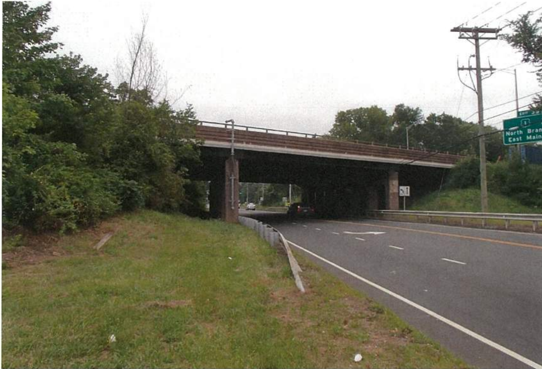
1. North Elevation (Note: View is looking Southbound on Route 1)
