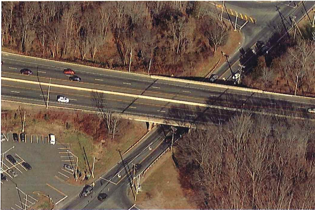
Image 1: Bridge #00196. Image courtesy of Bing Maps.
