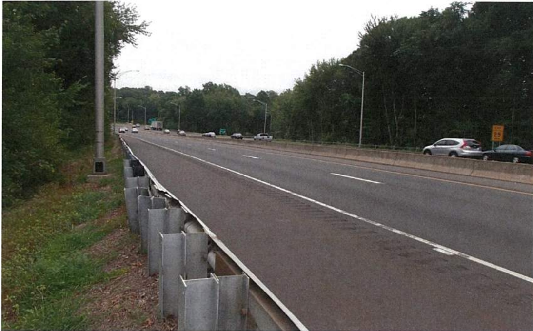
3. Southbound Lanes Looking East at East Approach
