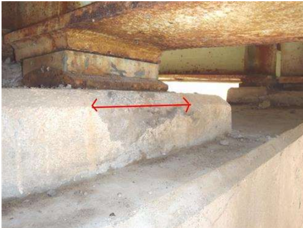
Large spall pedestal 3 pier 1, span 2 east side.
