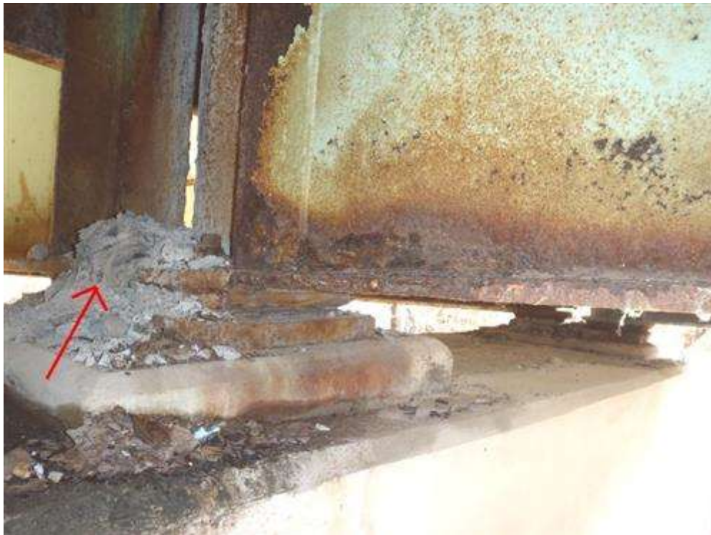
Pier 2, concrete between beam ends.
