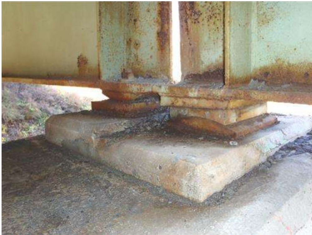
Typical bearings pier 1.
