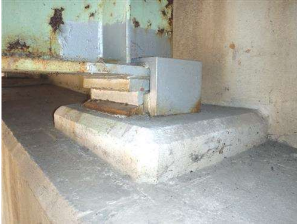
Typical expansion bearing east abutment
