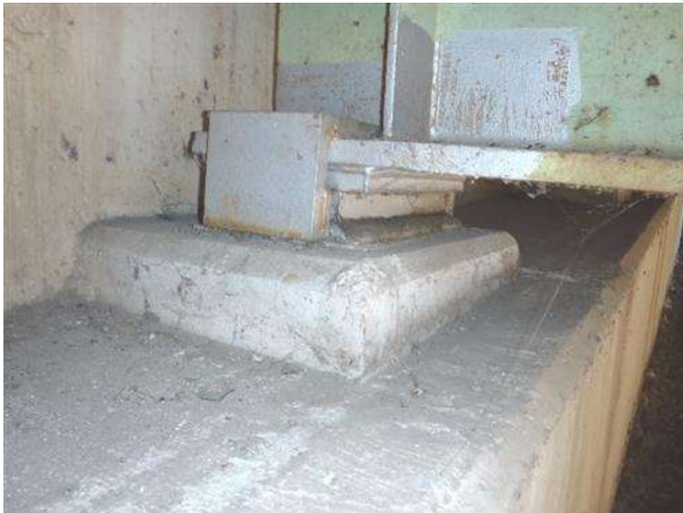
Typical expansion bearing west abutment.
