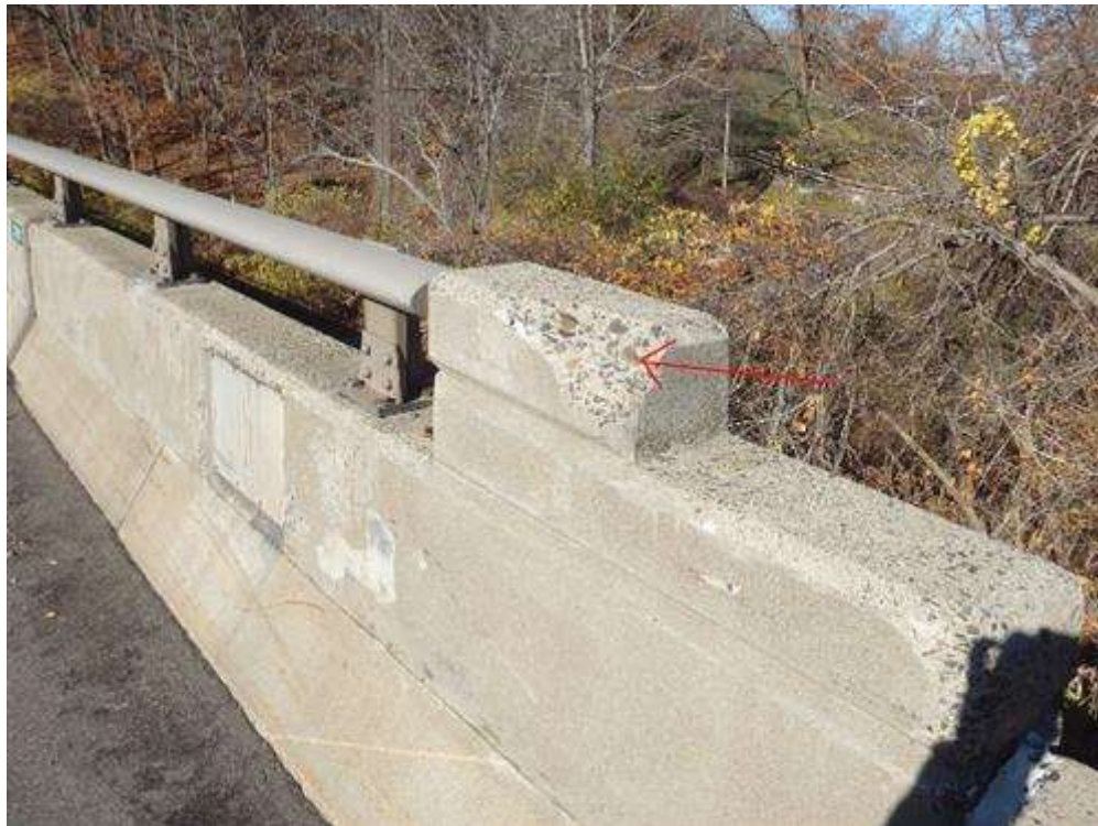
Large spall at approach parapet northeast corner.
