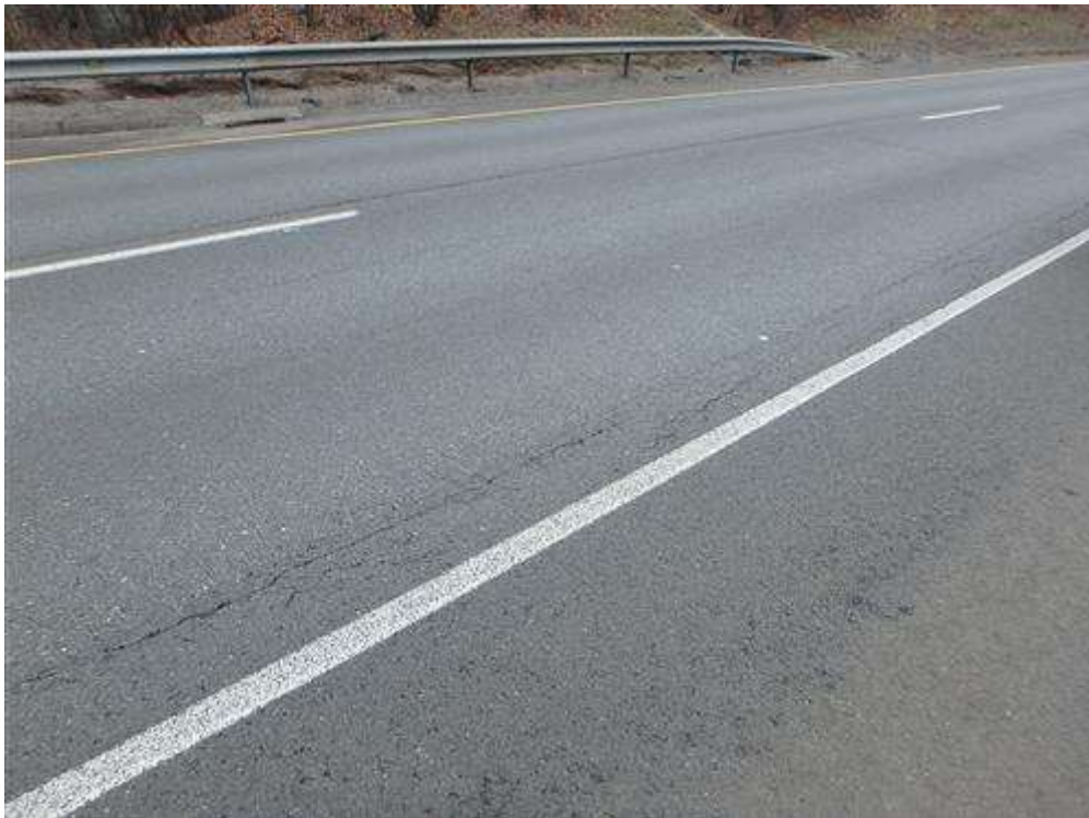
East approach bituminous pavement. Typical condition with open paving seams.
