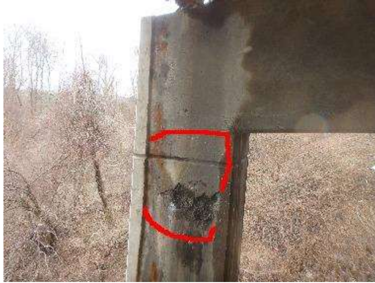
Pier 1, Column 4, east side, has a hollow area with spall.
