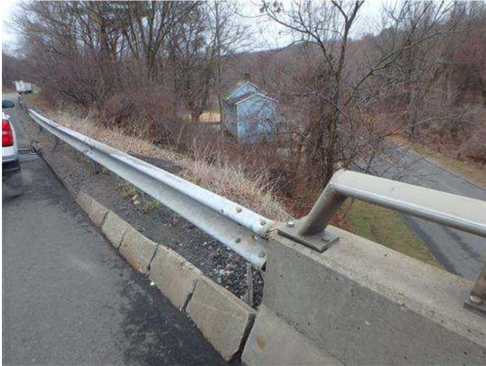
Southeast metal beam guide rail (trailing end). Typical condition.
