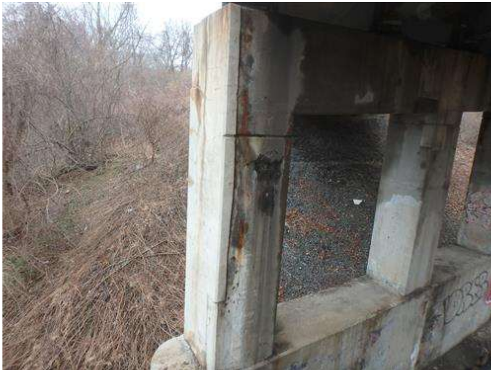
Same location as previous photo. Concrete patch on the south side of cap and column has hairline map cracks.
