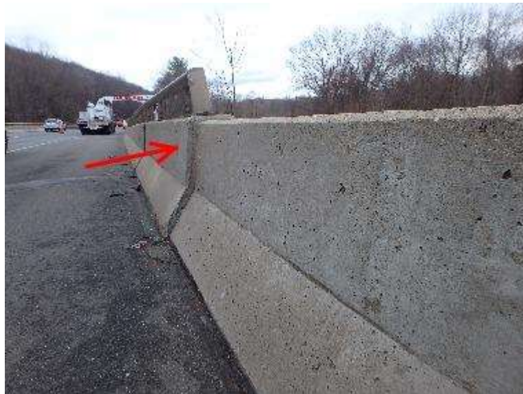
Southwest approach jersey barrier is laterally misaligned with the end of the wingwall parapet.
