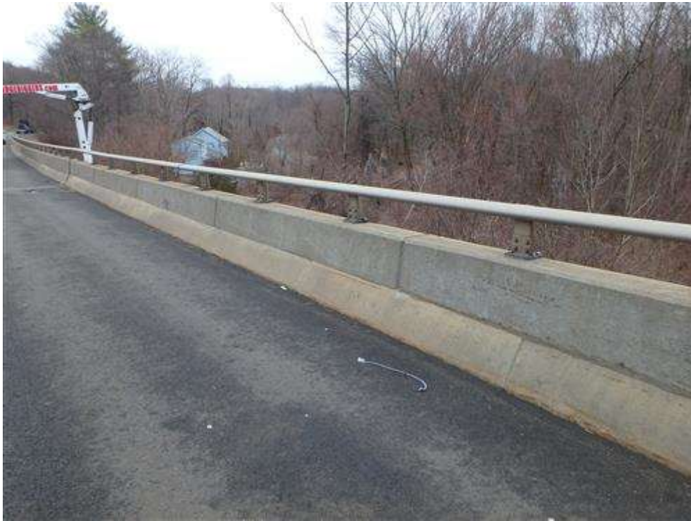
Typical curb, parapet and bridge railing condition. South side shown.
