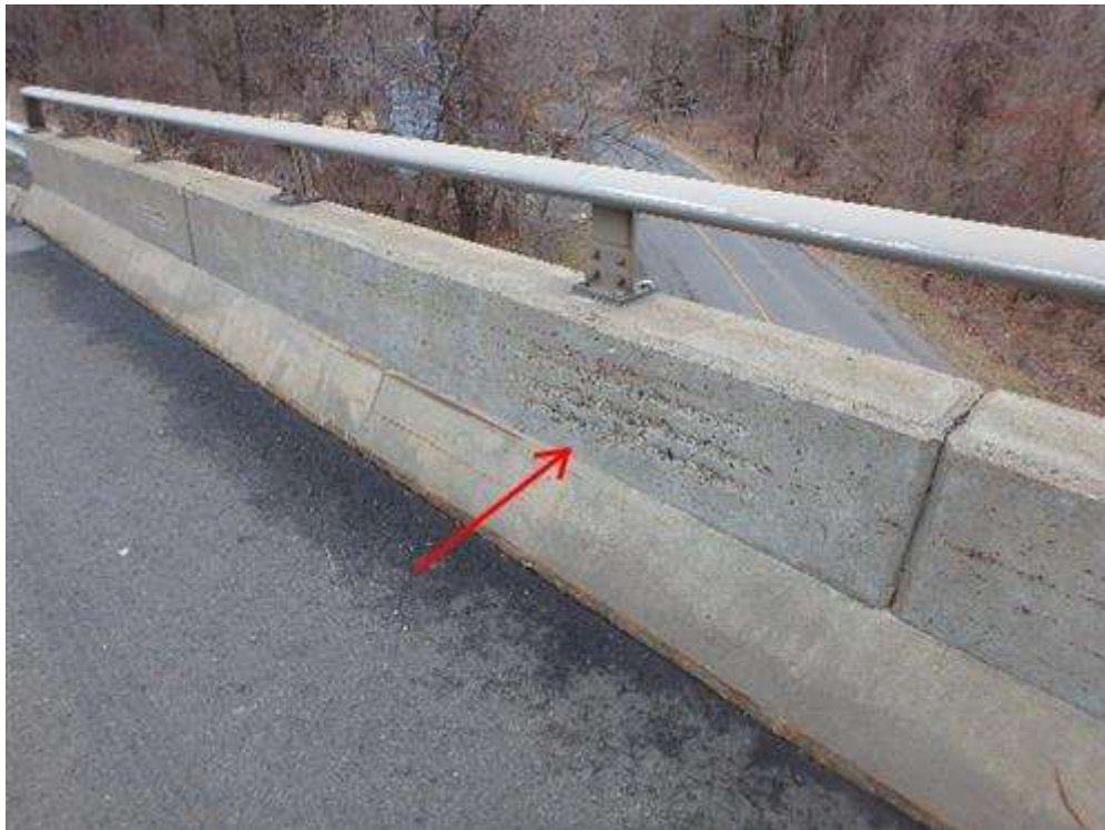
Span 3, south parapet has impact scrapes near mid-span.
