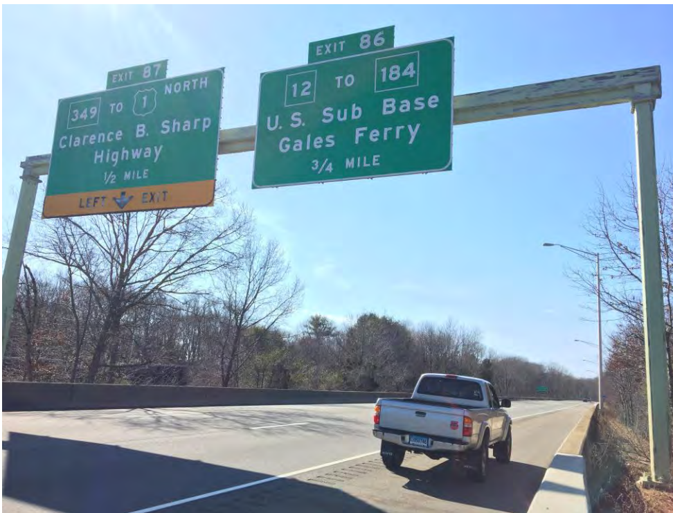
PHOTO 14 Site No. 15 – Sign Support No. 21210
