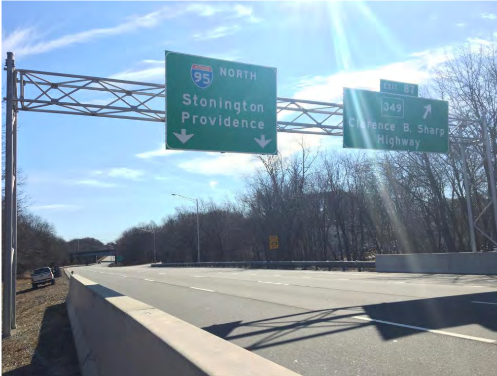
PHOTO 5 Site No. 5 – Sign Support No. 21198
