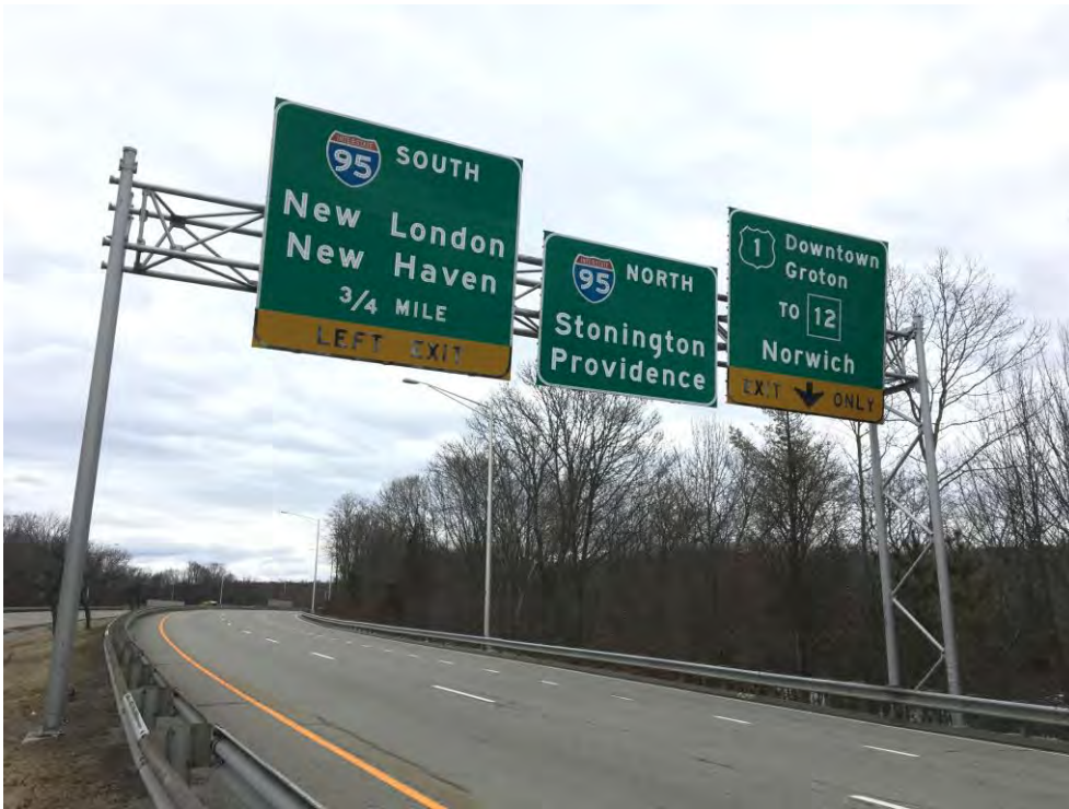
PHOTO 18 Site No. 19 – Sign Support No. 21291
