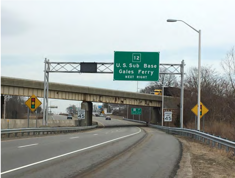
PHOTO 3 Site No. 3 – Sign Support No. 21195
