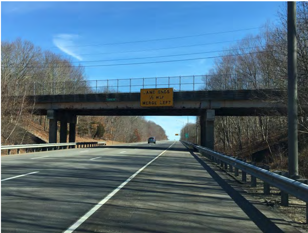
PHOTO 6 Site No. 6 – Sign Support No. 21199
