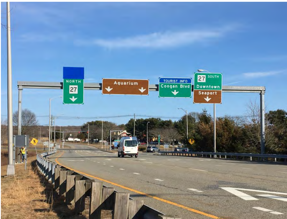
PHOTO 12 Site No. 13 – Sign Support No. 21206
