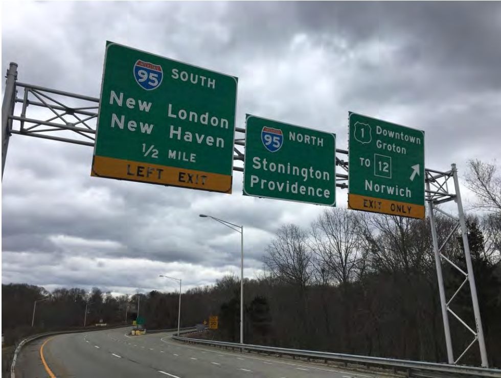
PHOTO 19 Site No. 20 – Sign Support No. 21292
