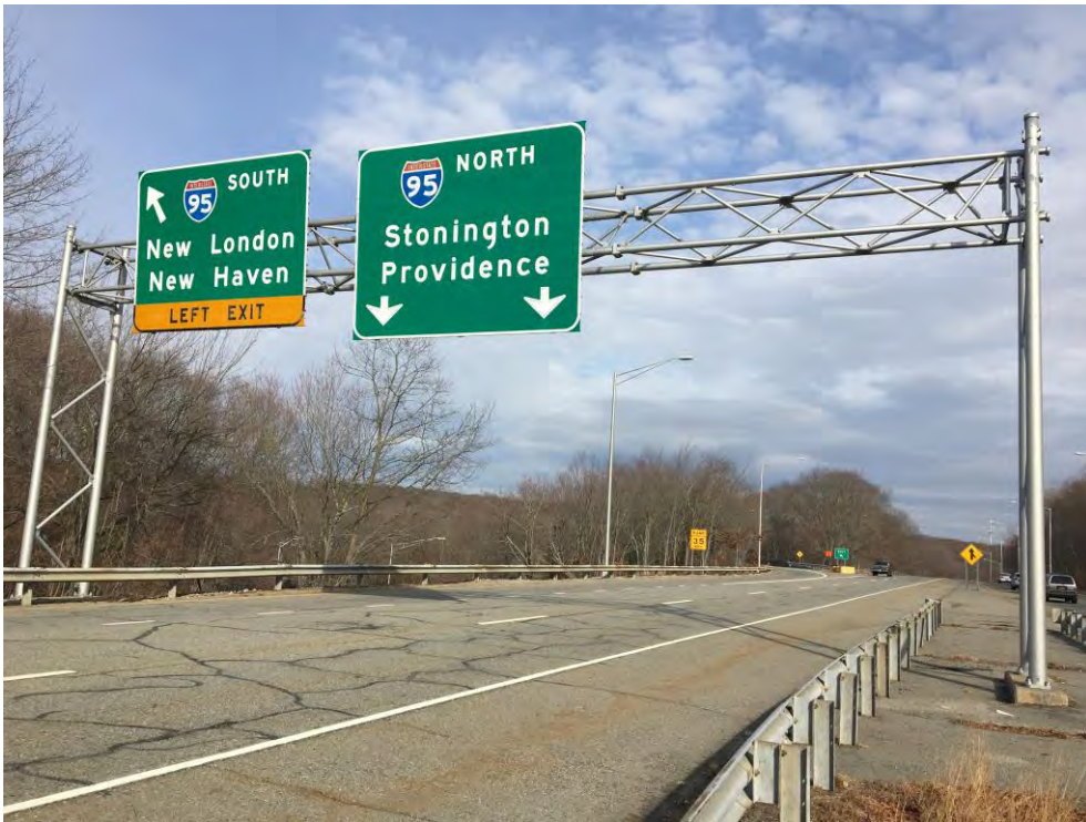
PHOTO 20 Site No. 21 – Sign Support No. 21293
