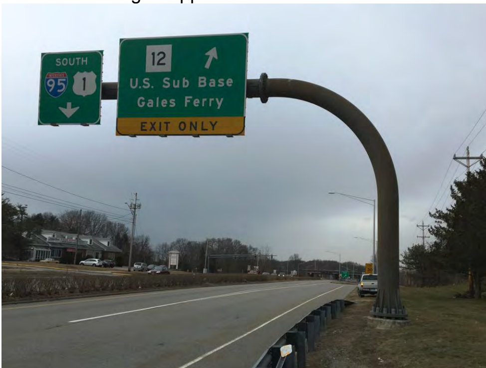
PHOTO 22 Site No. 23 – Sign Support No. 21954
