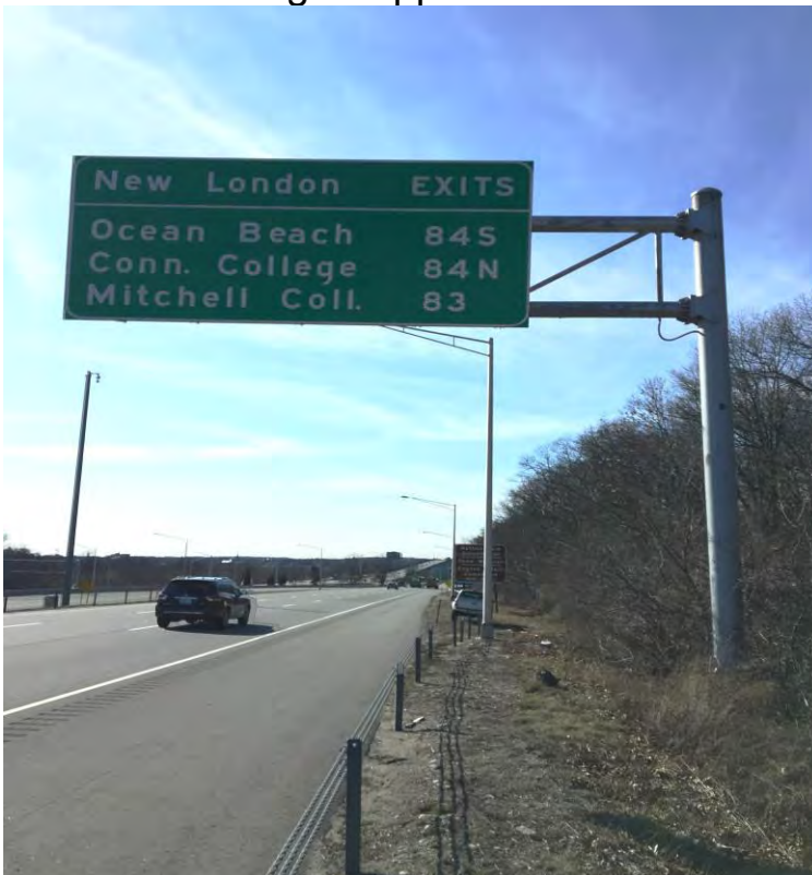
PHOTO 16 Site No. 17 – Sign Support No. 21214
