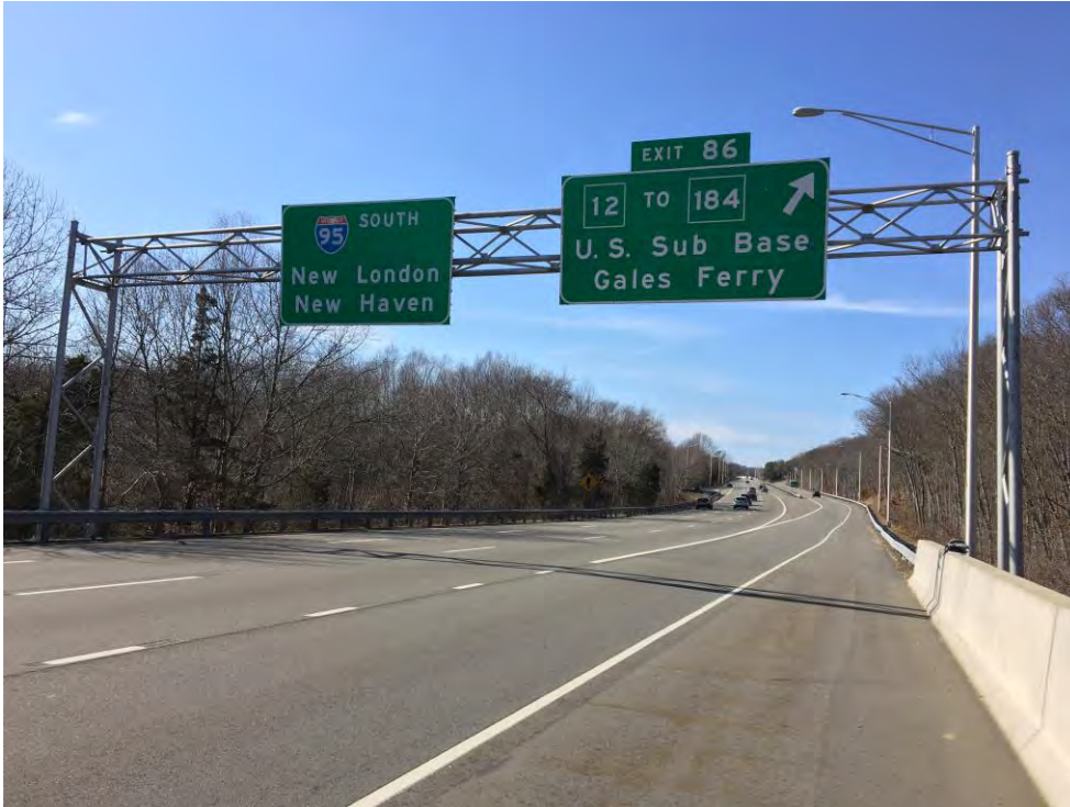
PHOTO 15 Site No. 16 – Sign Support No. 21212
