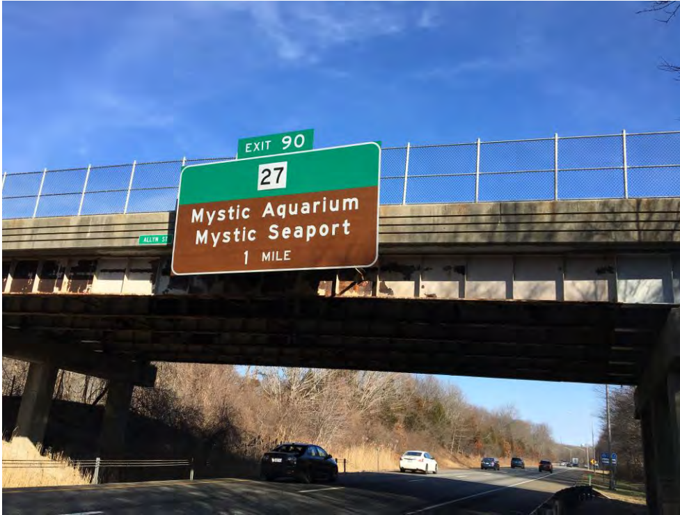
PHOTO 9 Site No. 10 – Sign Support No. 21203
