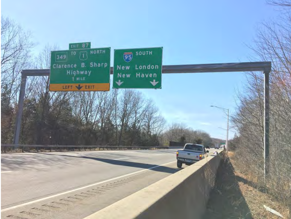
PHOTO 13 Site No. 14 – Sign Support No. 21209
