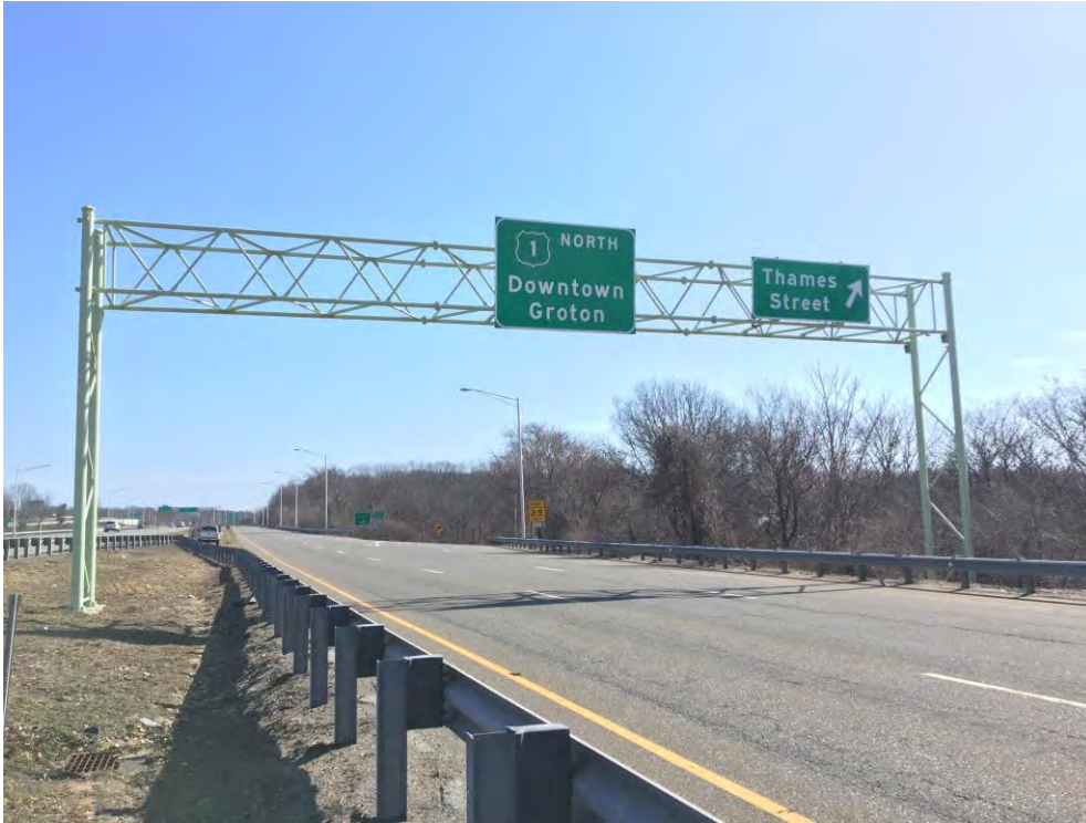
PHOTO 1 Site No. 1 – Sign Support No. 21193
