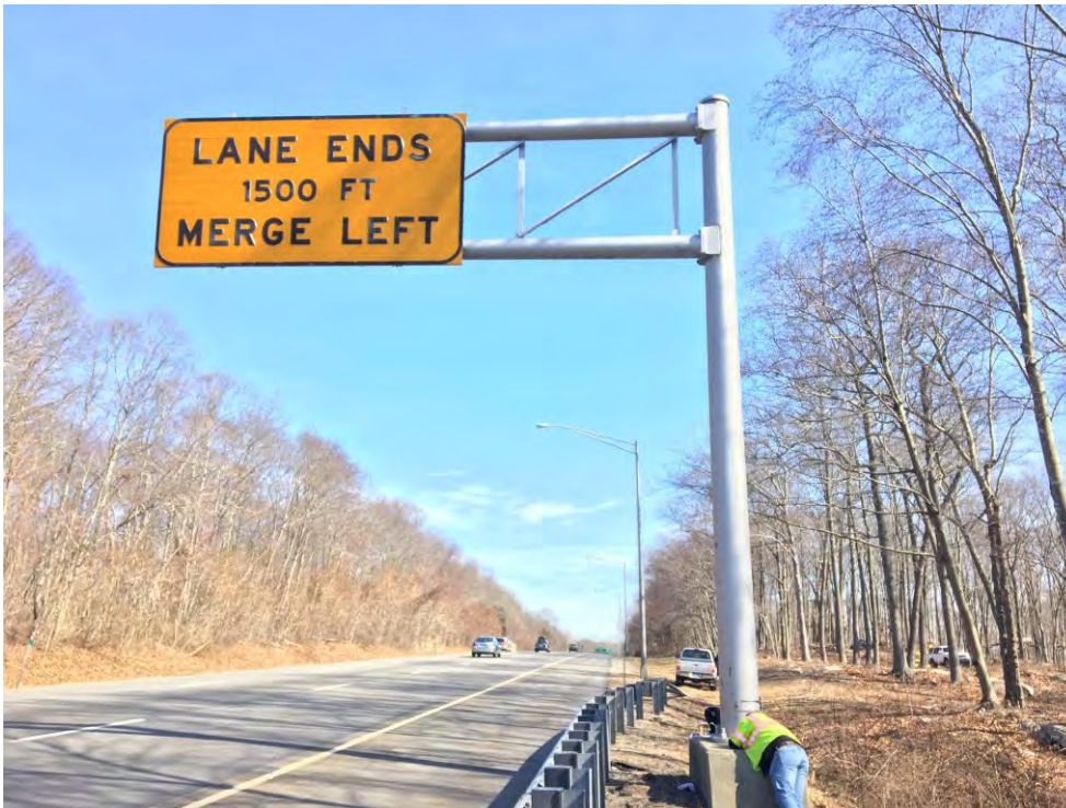
PHOTO 7 Site No. 7 – Sign Support No. 21200
