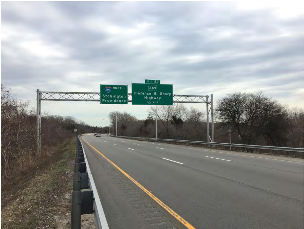
PHOTO 4 Site No. 4 – Sign Support No. 21197
