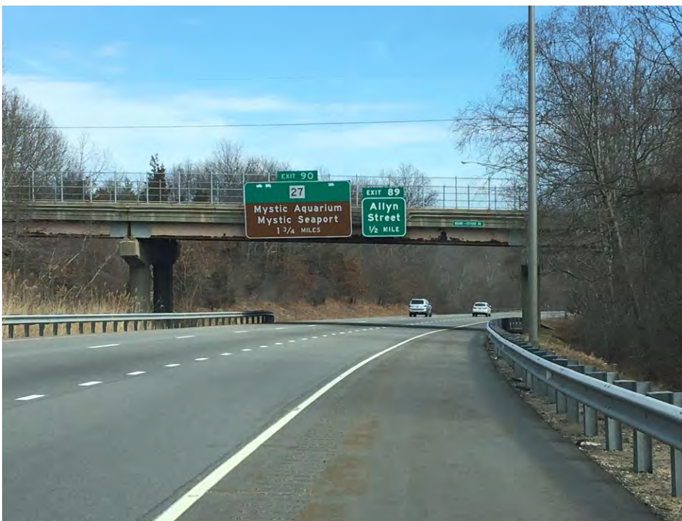
PHOTO 8 Site No. 8/9 – Sign Support Nos. 21201A & 21201B
