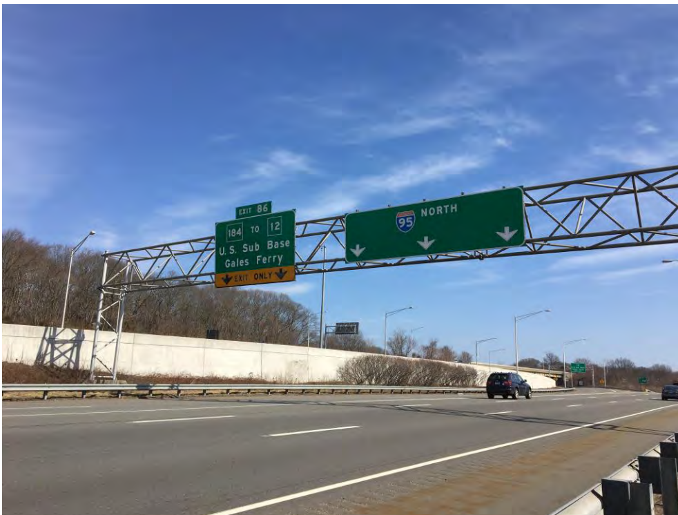
PHOTO 2 Site No. 2 – Sign Support No. 21194
