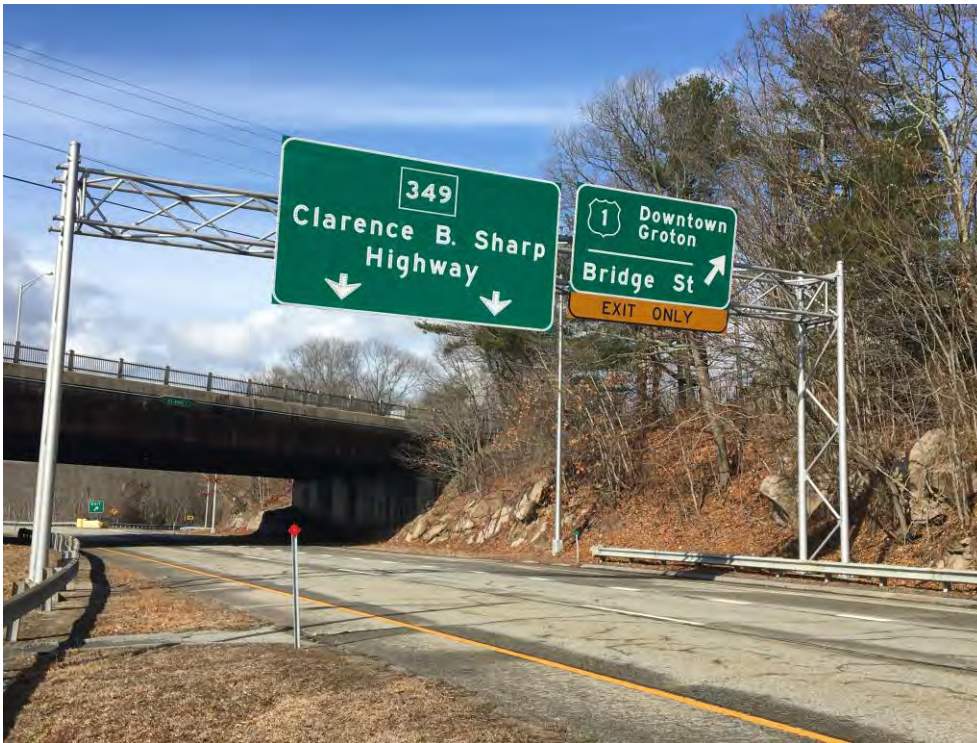
PHOTO 17 Site No. 18 – Sign Support No. 21288
