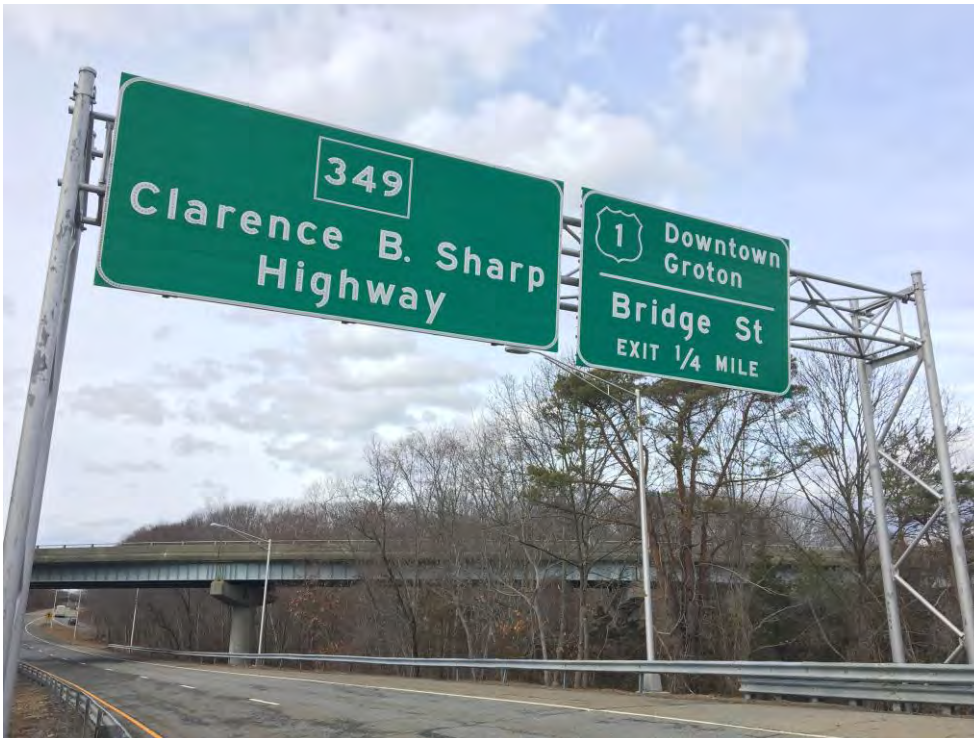
PHOTO 21 Site No. 22 – Sign Support No. 21294
