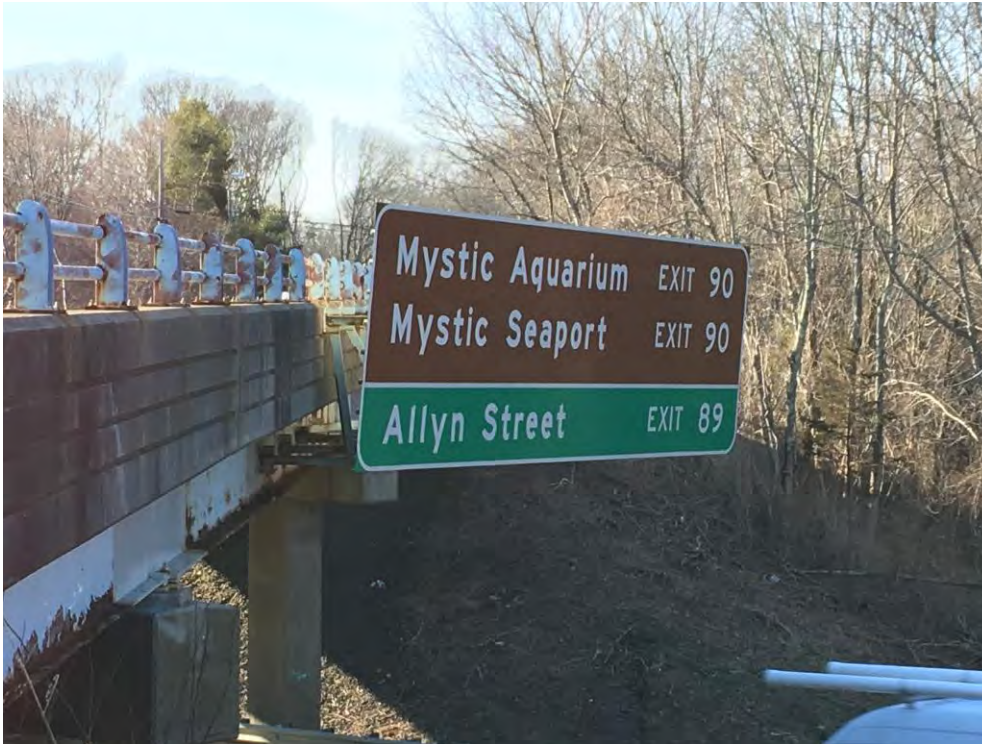
PHOTO 11 Site No. 12 – Sign Support No. 21205
