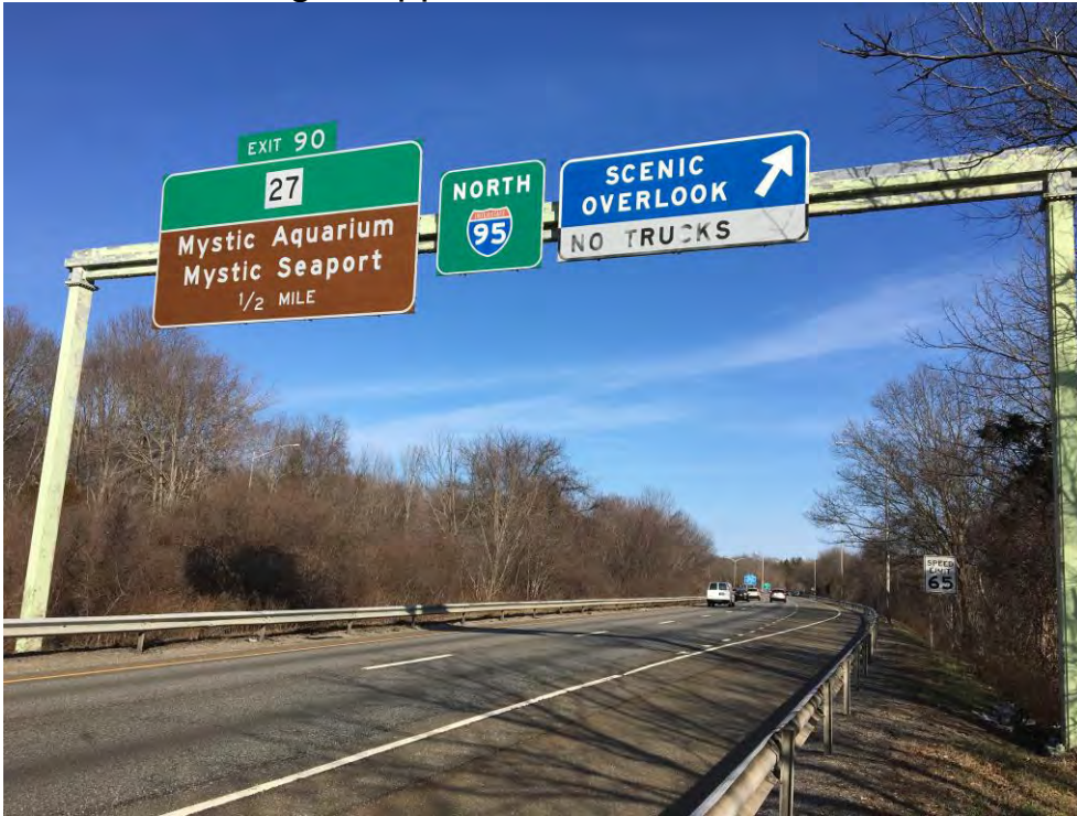
PHOTO 10 Site No. 11 – Sign Support No. 21204
