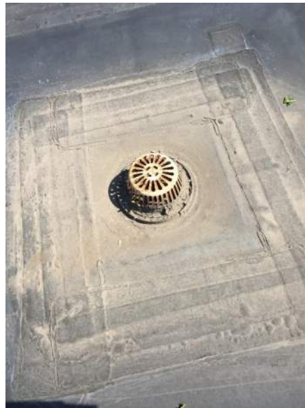
Existing Roof Drain. Typical.
