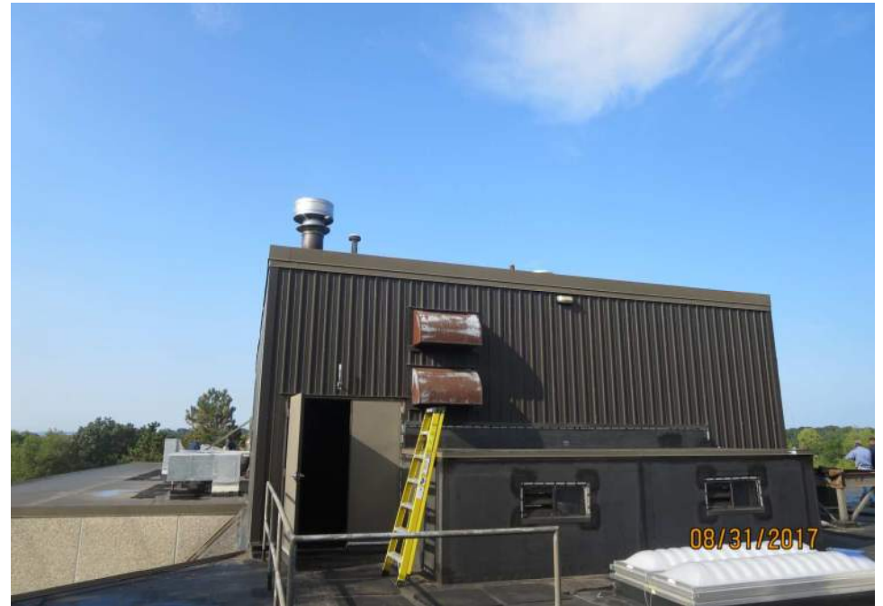
Mechanical Penthouse with Elevator Penthouse in front
