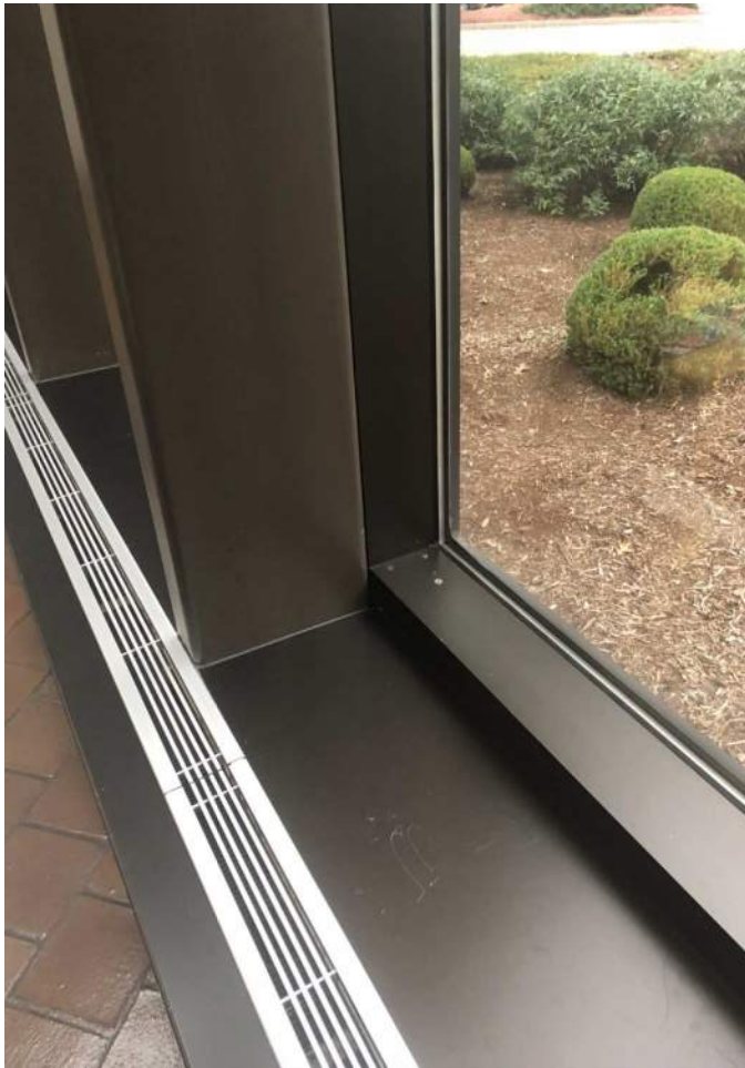
Interior at Sloped Glazing
