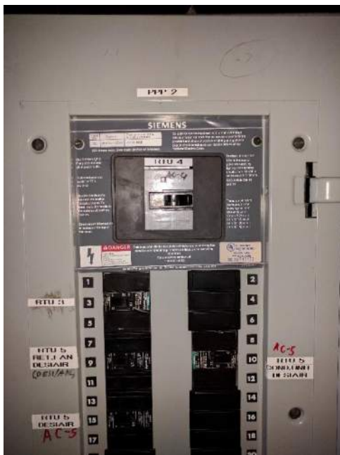
Existing Penthouse PP2
