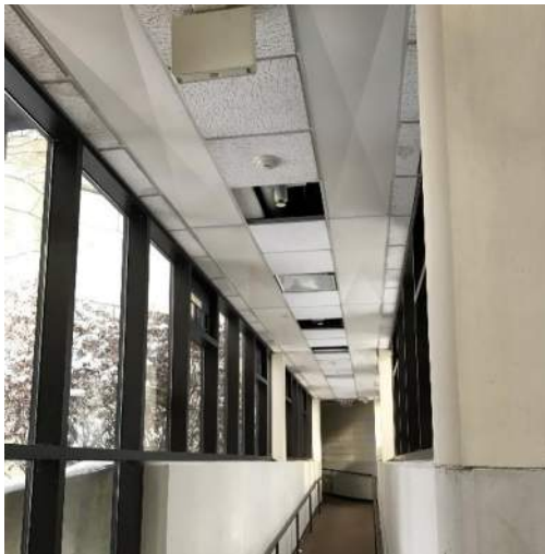
Existing Fire Protection & Radiant Panels in Connector
