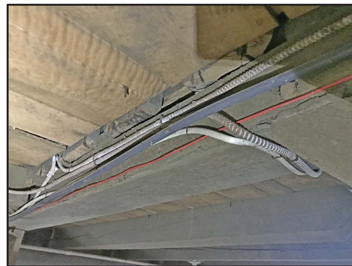
P03 FIRST FLOOR WALL PLANK VISIBLE IN BASEMENT DUE TO DEFLECTIONS. INSTALL NEW BLOCKING TIGHT TO UNDERSIDE OF PLANKS AND SHIM AS NEEDED. SEE DETAIL. REMOVE AND REINSTALL WIRING AS NEEDED.
