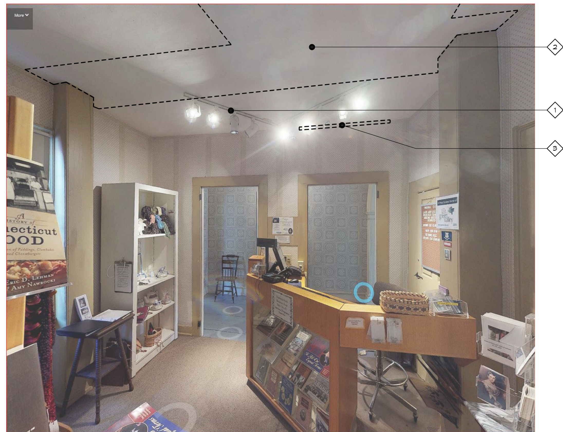
15 ROOM 113 NORTH PHOTOGRAPH NO SCALE
