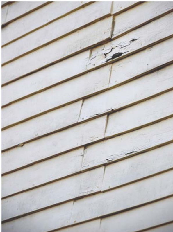
PHOTO 16 Zippered clapboard installation.
