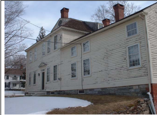
Photo C-1-9: Electric service meter and telephone feed
