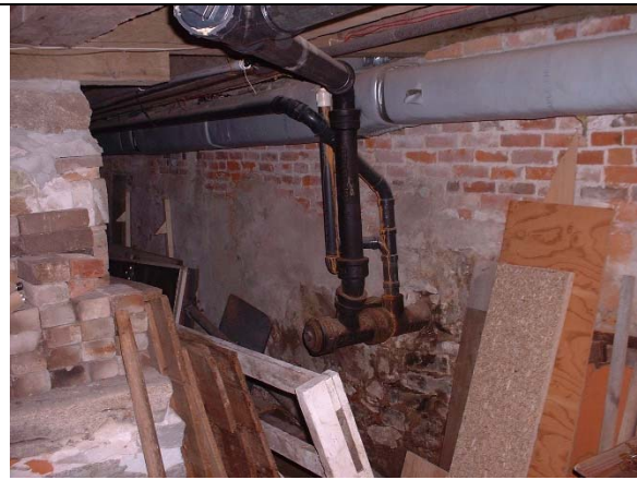
Photo C-1-6: Sanitary sewer piping exiting through foundation wall
