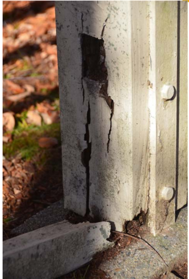
PHOTO 69 Steel brackets embedded in concrete.
