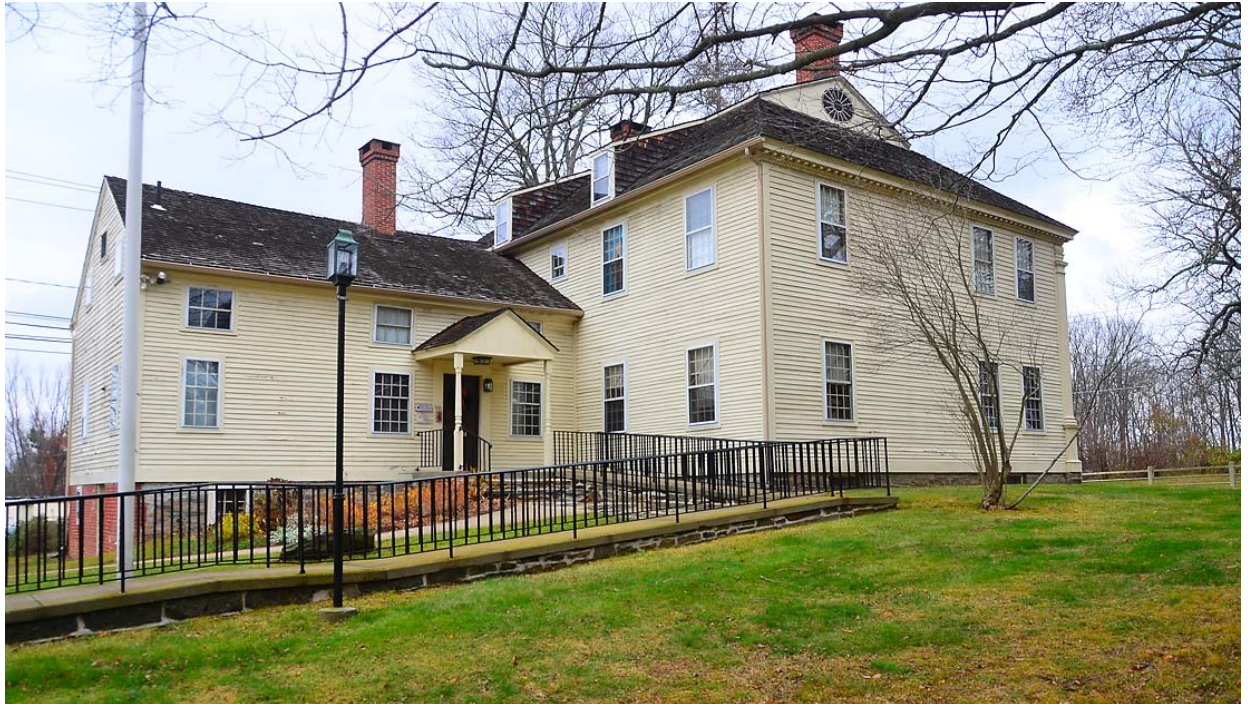
View from the southwest and the Carter House rear yard.
