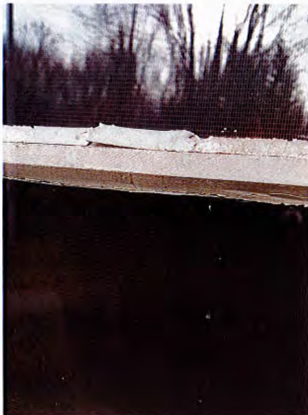
Exterior window glaze
