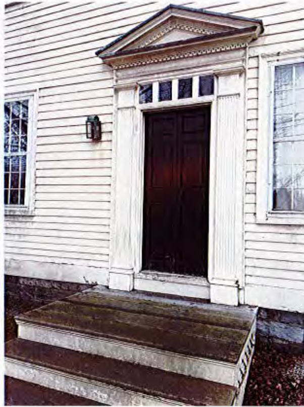
Street side door outside of foyer
