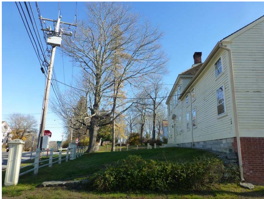
Photo C-2-18: Incoming electrical service
