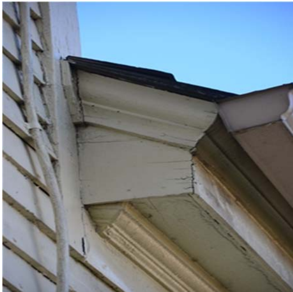
PHOTO 21 Eave at Ell.
