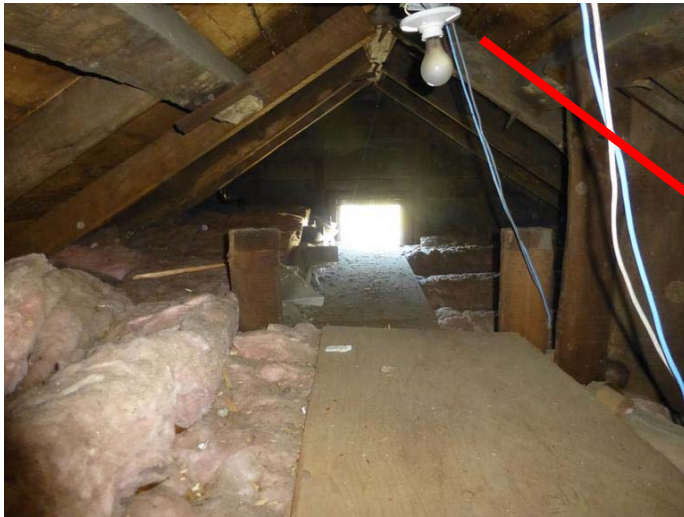
Photo C-2-15: Attic above Ell
