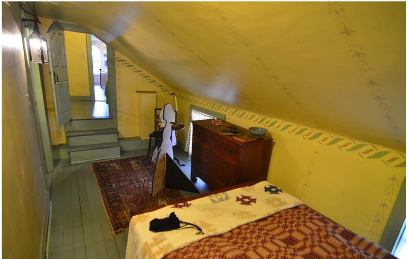
PHOTO 83 Uninsulated roof contributes to significant ice dams over Ell entrance on south wall.
