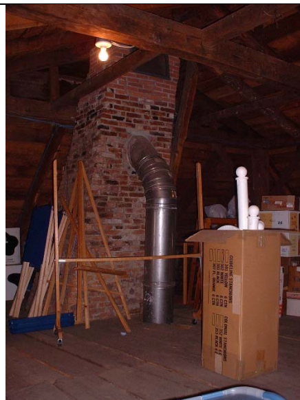
Photo C-1-8: Boiler flue connection to chimney in attic
