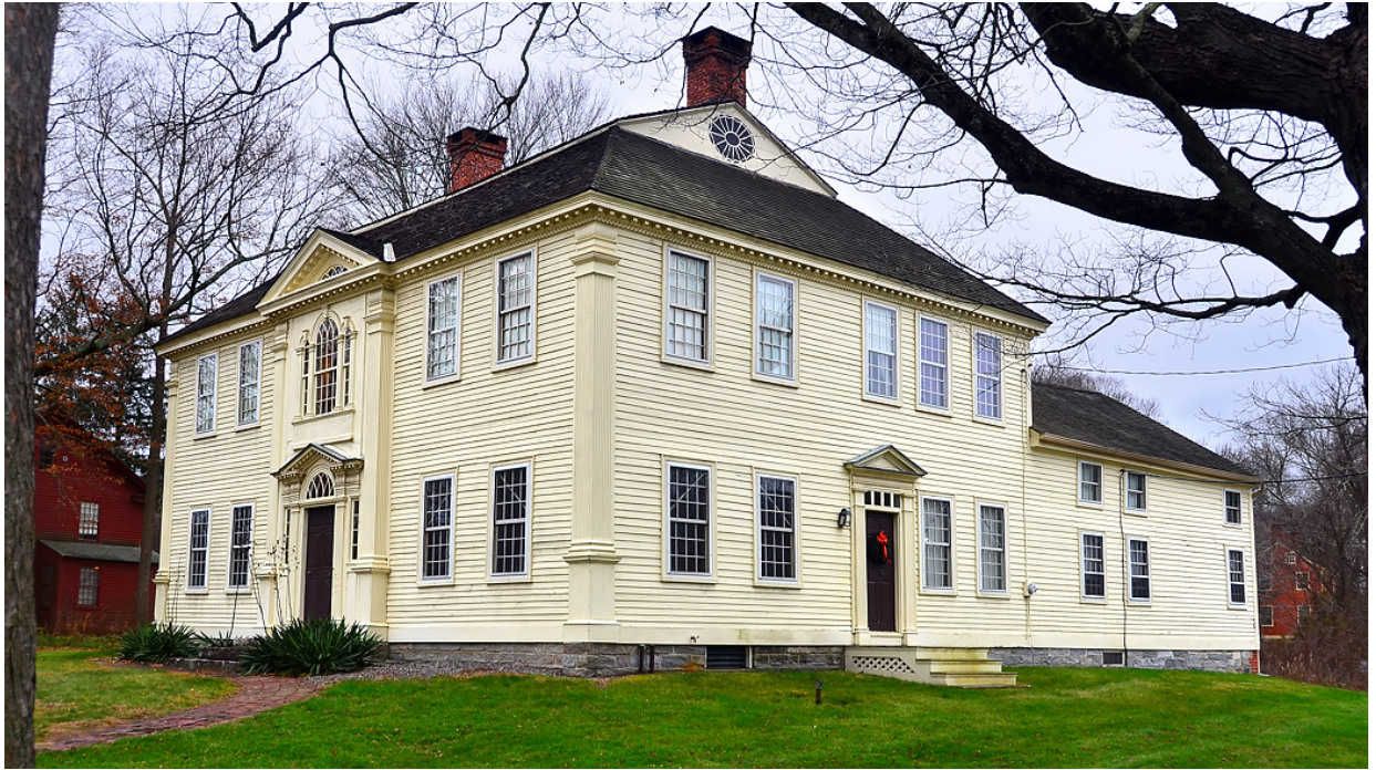
View from northeast: Intersection of Westminster Road and South Canterbury Road
