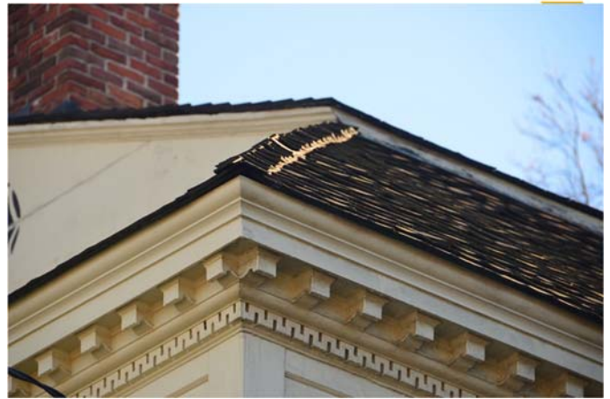
PHOTO 17 Cornice decorative trim in good shape.
