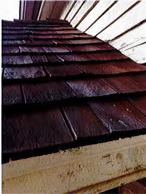
Clapboard Roof
