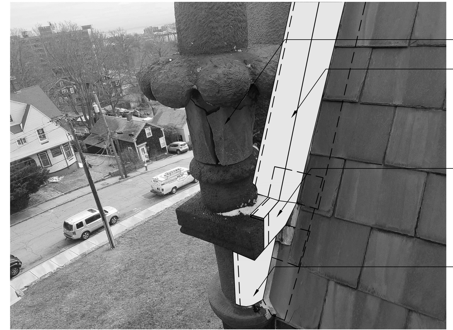
6 PHOTO: ROOF TO POST BASE FLASHING SCALE: NO SCALE
