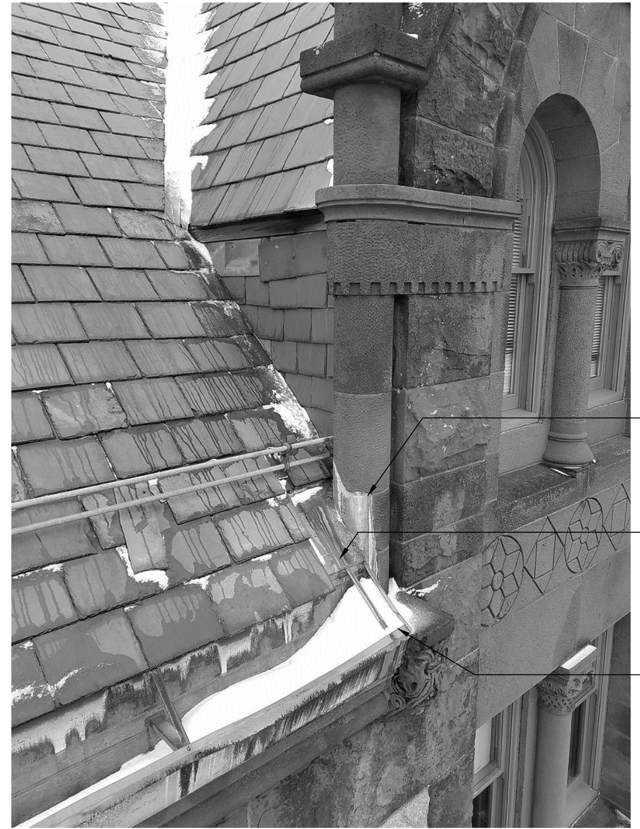
5 PHOTO: ROOF TO STONE POST FLASHING SCALE: NO SCALE
