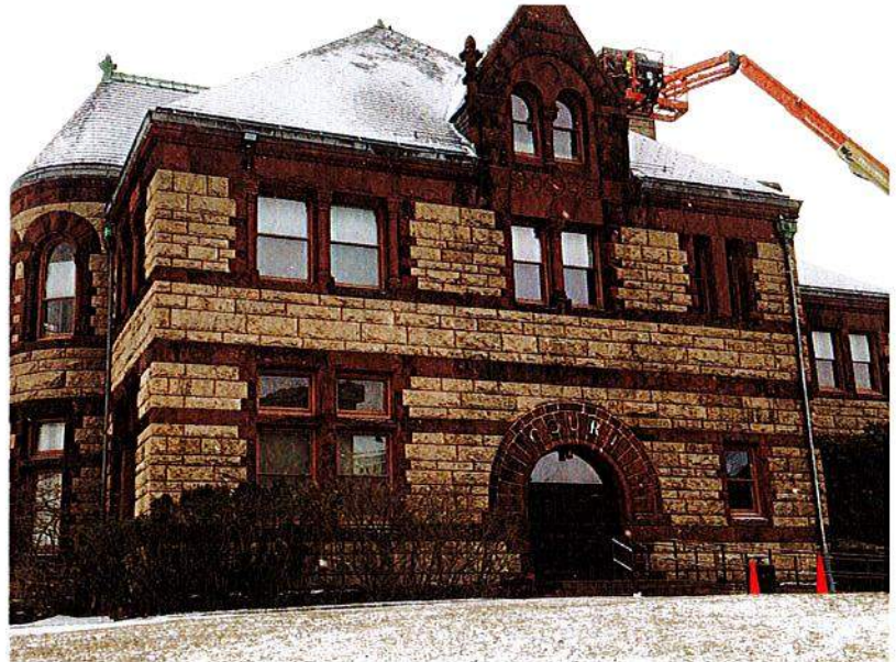
Exterior A side and D side downspouts. All the downspouts are galvanized.
