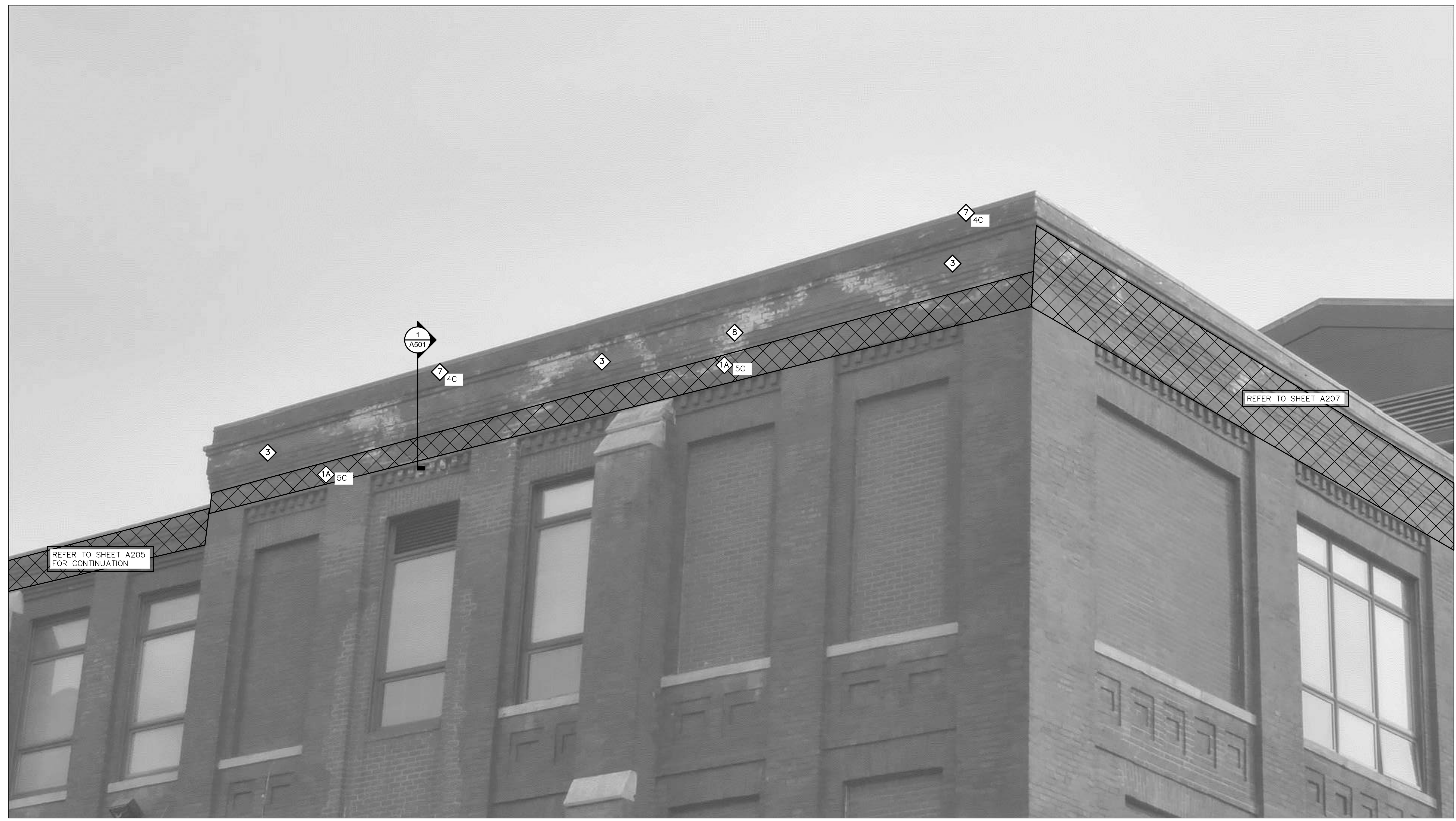
1 460 PHOTO ELEVATION - PARTIAL WEST MASONRY WORK SCALE: NOT TO SCALE
