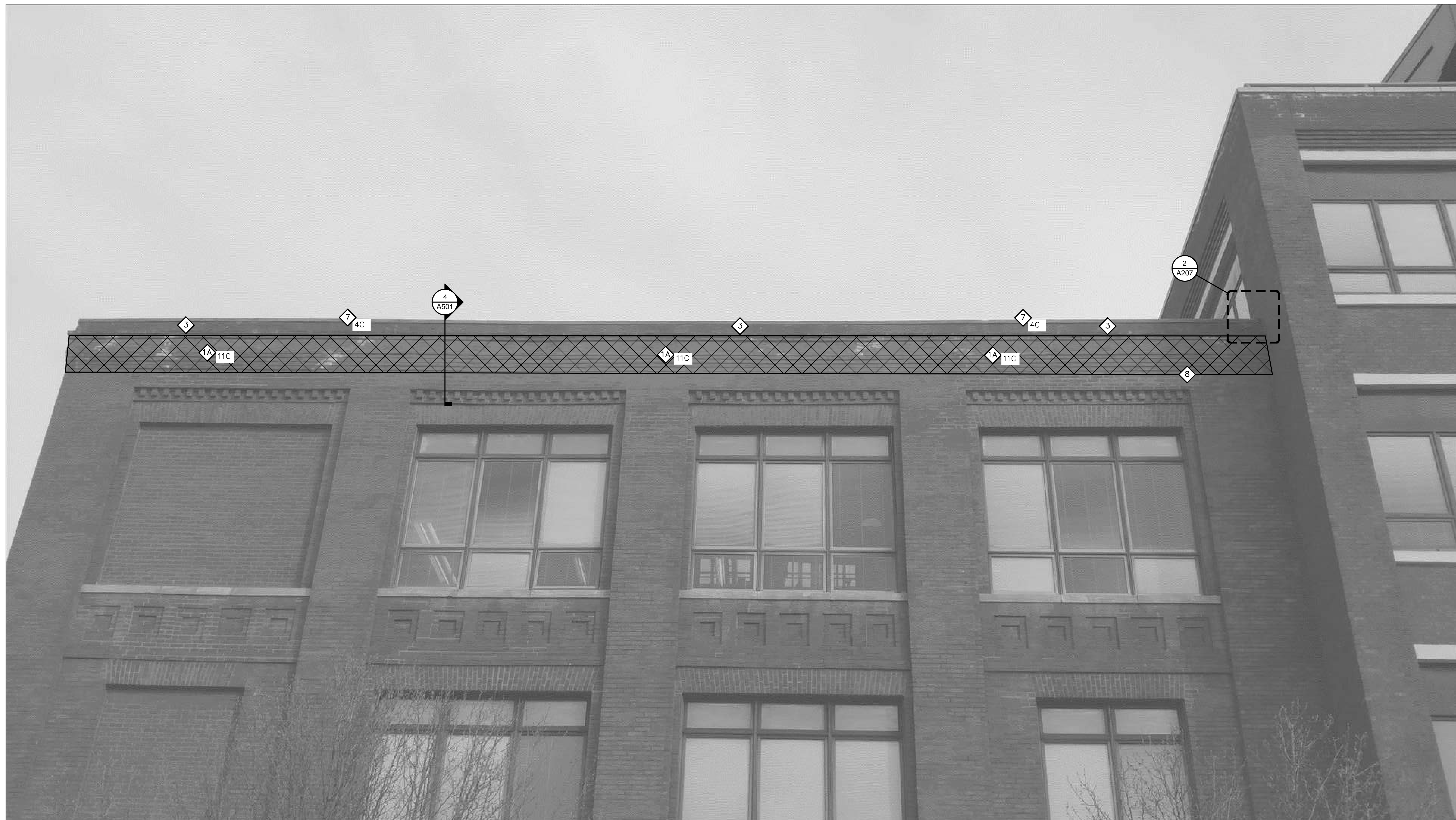
1 460 PHOTO ELEVATION – PARTIAL SOUTH MASONRY WORK SCALE: NOT TO SCALE
