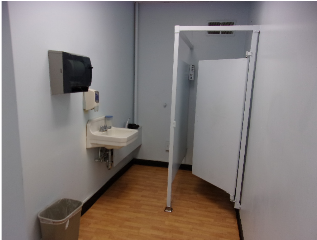
Building 2 - 2 nd floor woman's bathroom with wood grain laminate flooring over 12" x12" tan ACM floor tile
