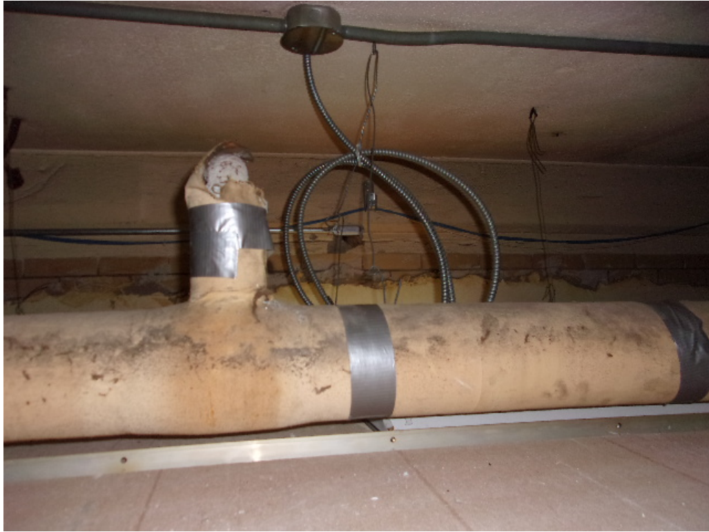
Building 2 - 2 nd floor woman's bathroom overhead ACM pipe and fitting insulation
