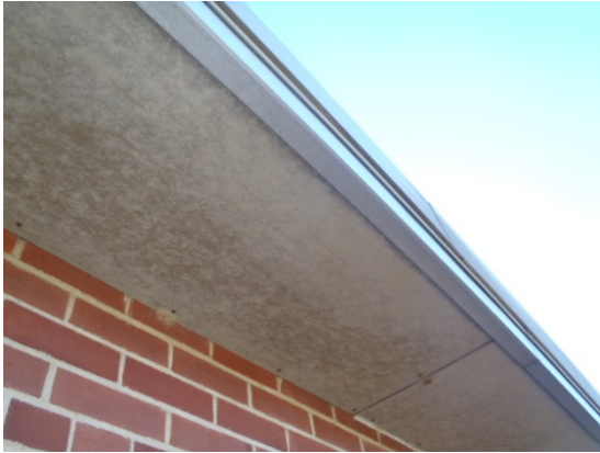
Student Center – Upper Roof (1) ACM Cementitious Soffit Paneling
