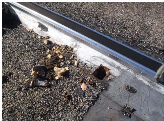
Student Center – Lower Roof (2) ACM Black Layered Roofing at Edge
