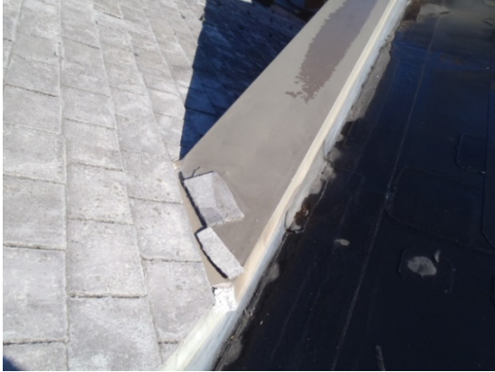
Theatre Roof – ACM Cementitious Roof Shingles on Adjacent Pitch Roof
