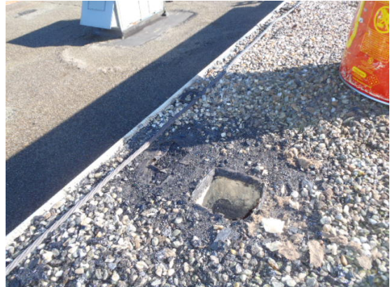
Student Center – Upper Roof (1) ACM Black Layered Roofing at Edge
