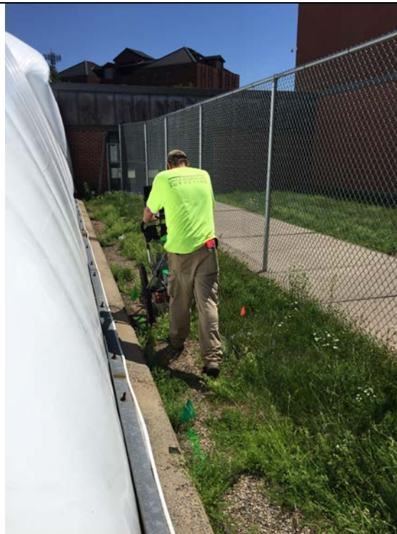
Photo 6: Underground Surveying performing underground utility mark-out near proposed location for SB-8. Sanitary sewer line located just north of the proposed boring
