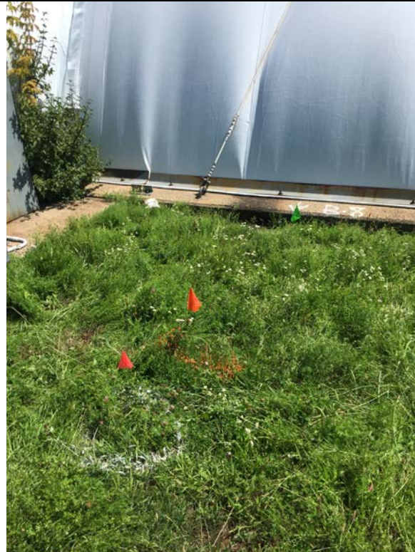
Photo 4: Communication and sanitary sewer lines located east of the proposed location for SB-6.
