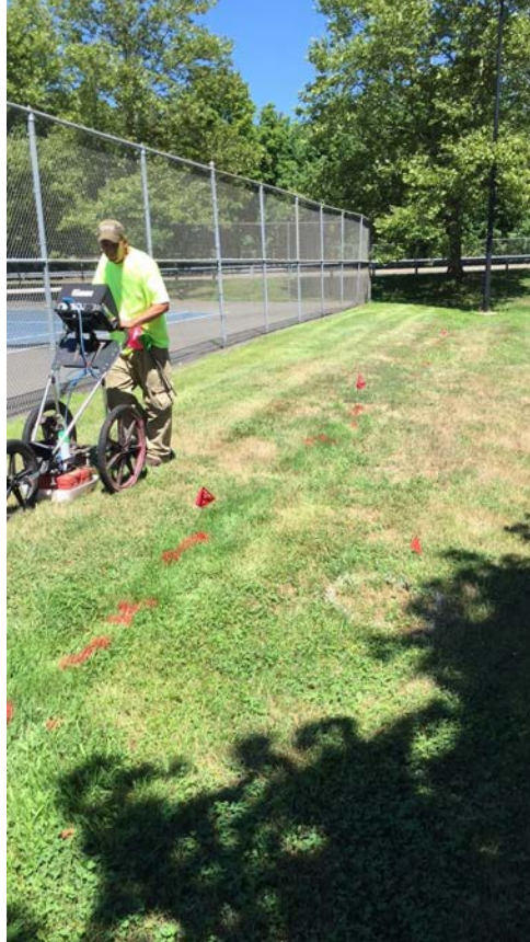
Photo 7: Underground Surveying performing underground utility mark-out near proposed location for SB-2. An electrical line is located just west of the proposed boring.
