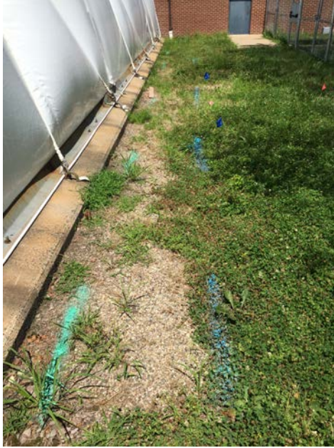
Photo 11: Sanitary sewer and water lines running north to south on the east side of the proposed location for SB-12.
