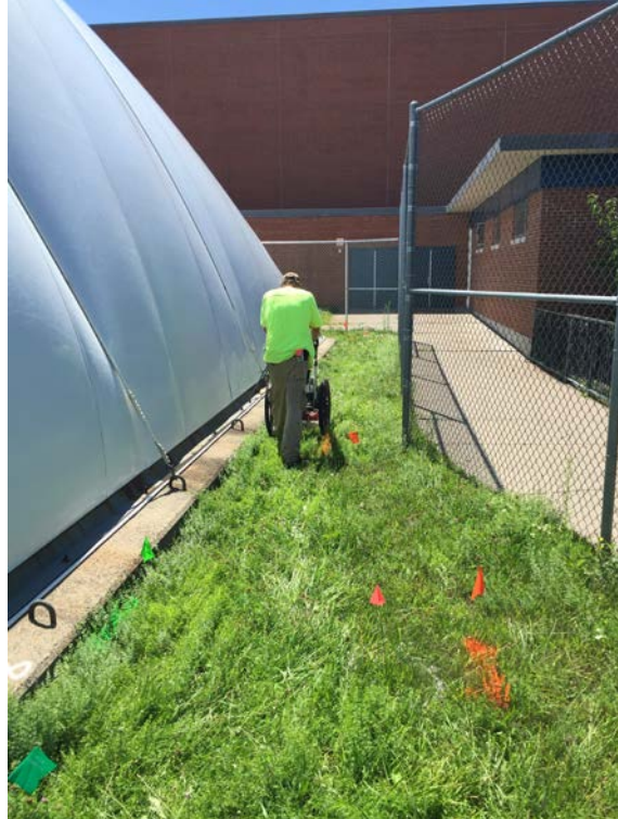
Photo 5: Underground Surveying performing underground utility mark-out near proposed location for SB-7. A communication line is located just west and a sanitary sewer line is located east of the proposed boring.
