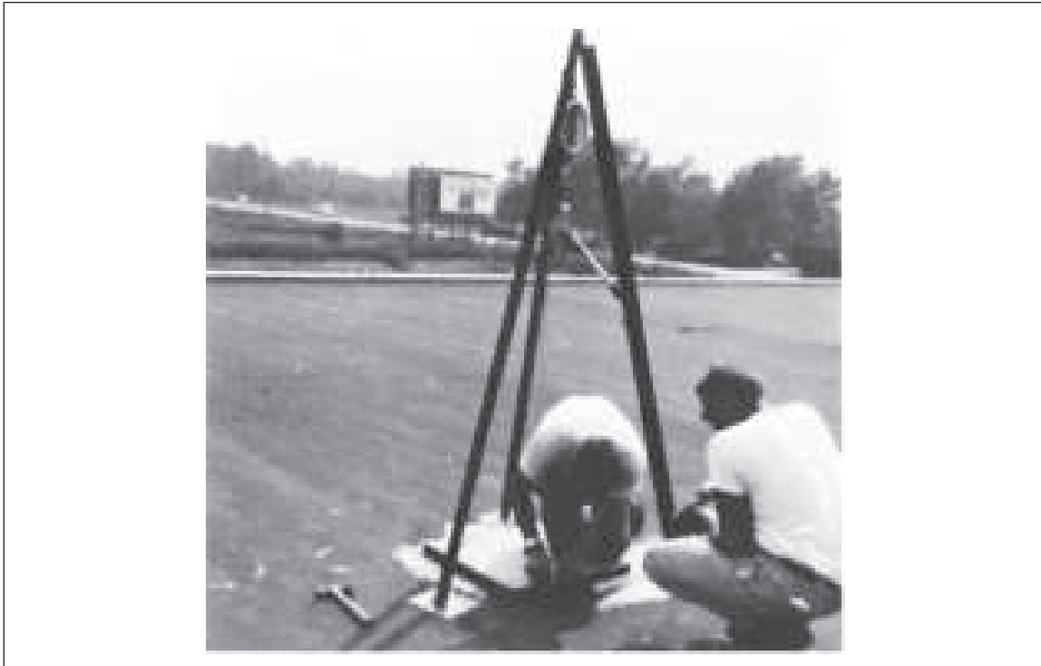
Fig. 7. Bonded uplift test
